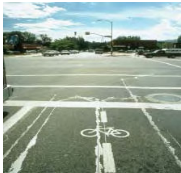
Pavement markings indicate to bicyclists where they should position themselves to activate the signal detector.
