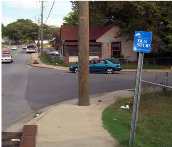
The pole in the sidewalk is an example of an obstruction that is non-compliant with ADA guidelines.
