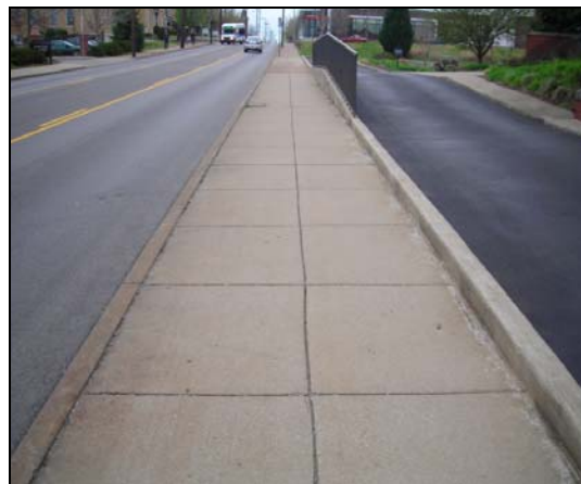
Figure 4-6. Example of "Good" Sidewalk Condition
