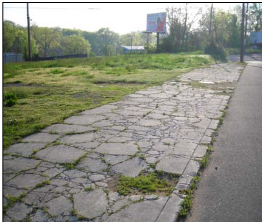
Figure 4-8. Example of “Poor” Sidewalk Condition
