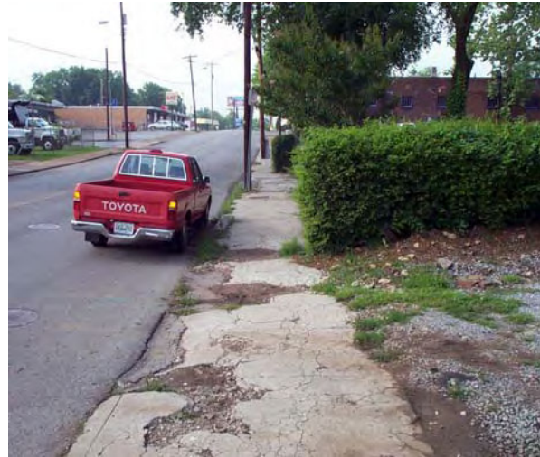
This sidewalk segment illustrates a damaged sidewalk, one of the various sidewalk problems identified by the inventory.
