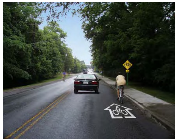
Shared roadways accommodate both vehicles and bicycles.
