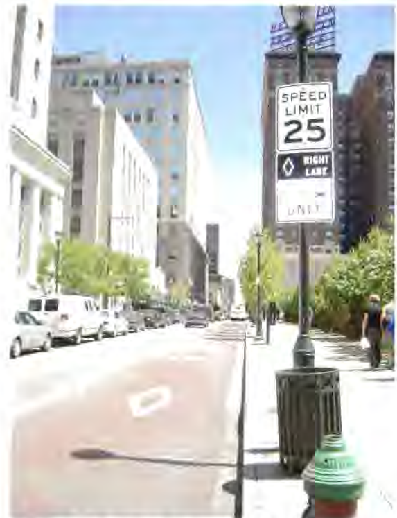
Shared bus/bike lanes, like this one in Philadelphia, can be a good alternative when there is not enough pavement width for separate bus and bike lanes.
