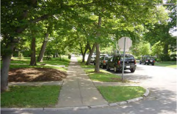
This corner is an example of a location that requires a sidewalk ramp per Metro standards and ADA guidelines.
