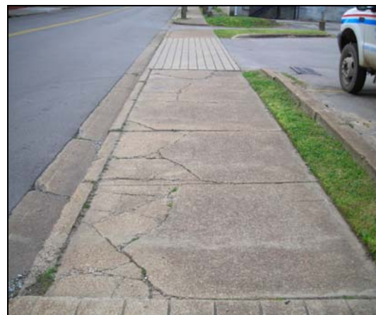
Figure 4-7. Example of "Fair" Sidewalk Condition
