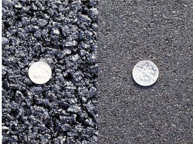
Figure C.4. NovaChip surface on the left; sand mix surface on the right.
