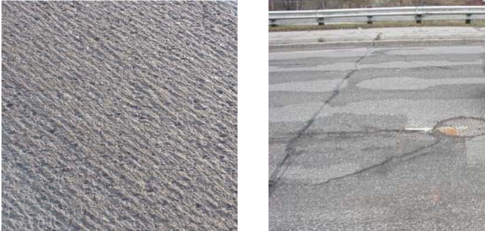
Figure C.18. Micro-milling application to reduce rutting and increase smoothness.
