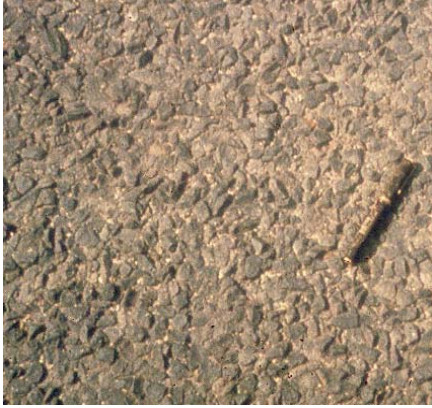
Figure C.12. Surface of a newly constructed surface treatment using uniform size aggregate.
