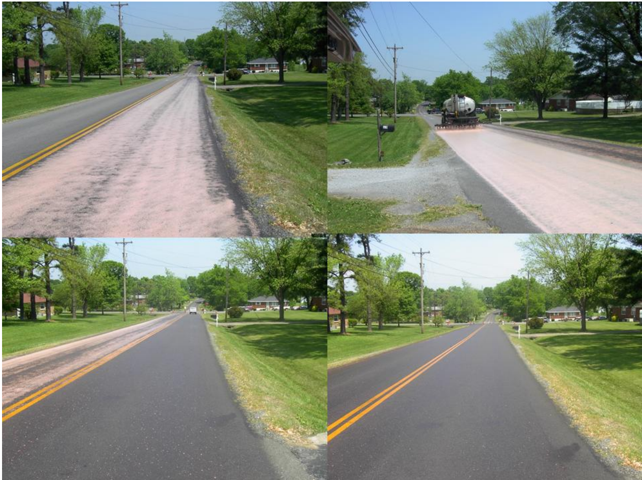
Figure C.20. Reclamite application on field section in Nashville.
