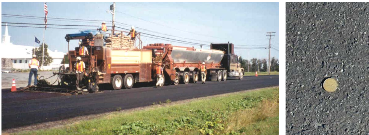
Figure C.7. Truck-mounted self-propelled micro-surfacing machine (left) and finished surface using Type II aggregate (right).
